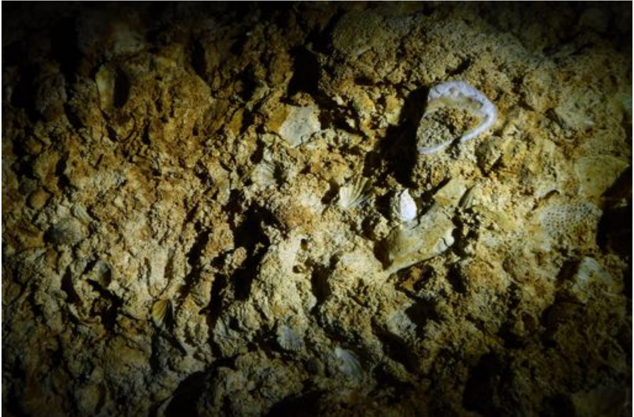
Fossilized ceiling! This was pretty cool to crawl under. Photo: Heather Duff
